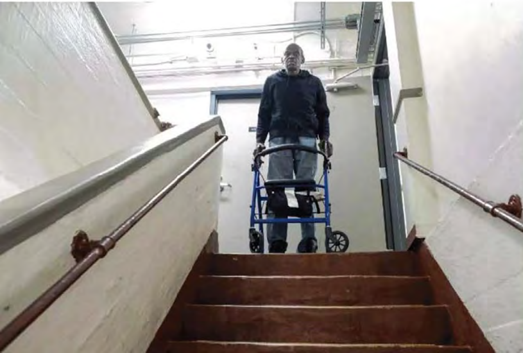
Kenneth Owens, 70, stands at the steps with his walker inside the Madison Hotel, which is owned by the AIDS Healthcare Foundation. Owens is one of 18 tenants who sued the foundation over a chronically broken elevator. (Francine Orr / Los Angeles Times)
