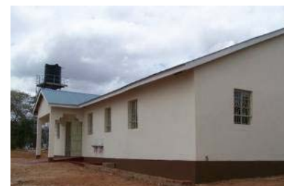
Kithituni Clinic after renovations
